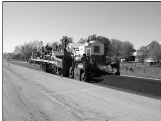
Figure 2. Cold In-place Recycled Expanded Asphalt Mix Train
