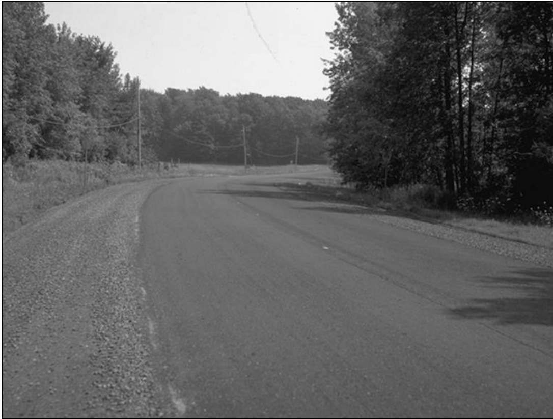
Figure 4. Emulsion Cold In-Place Recycling Project in Good Condition shortly after Construction
