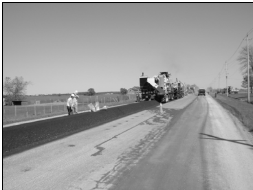
Figure 2. Cold In-place Recycled Expanded Asphalt Mix Train
