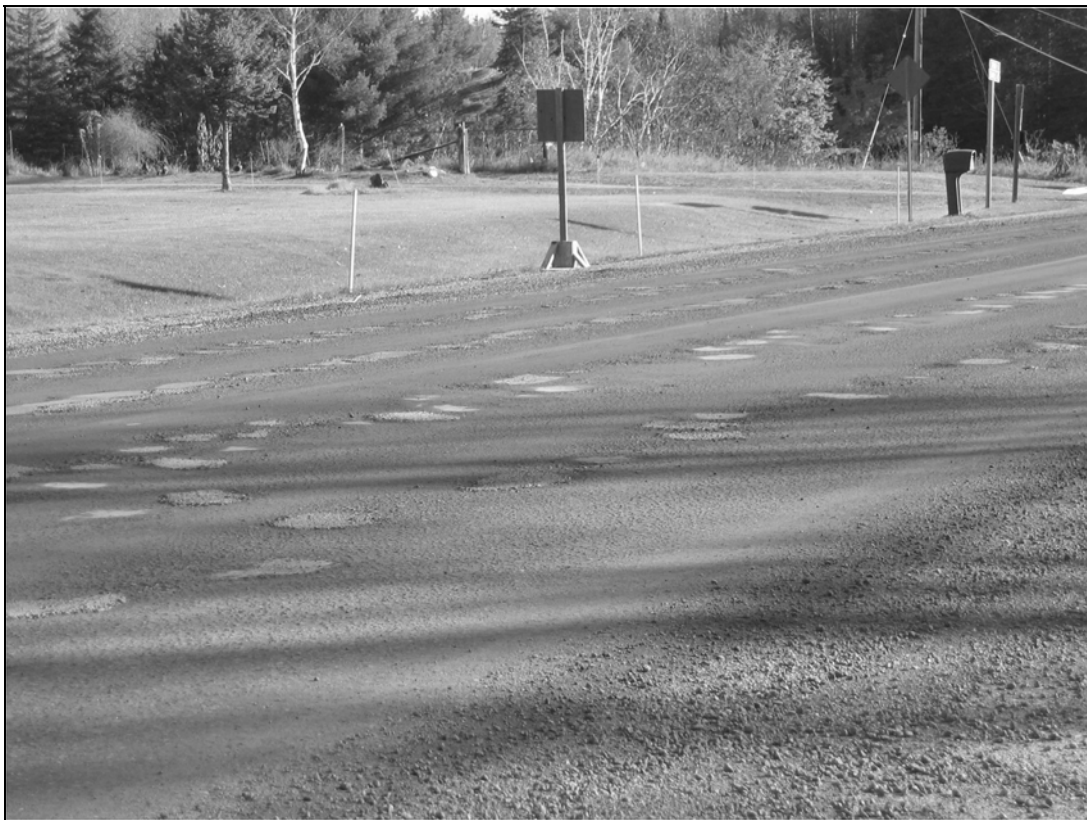
Figure 3. Cold In-place Recycled Expanded Asphalt Mix Failure shortly after Construction
